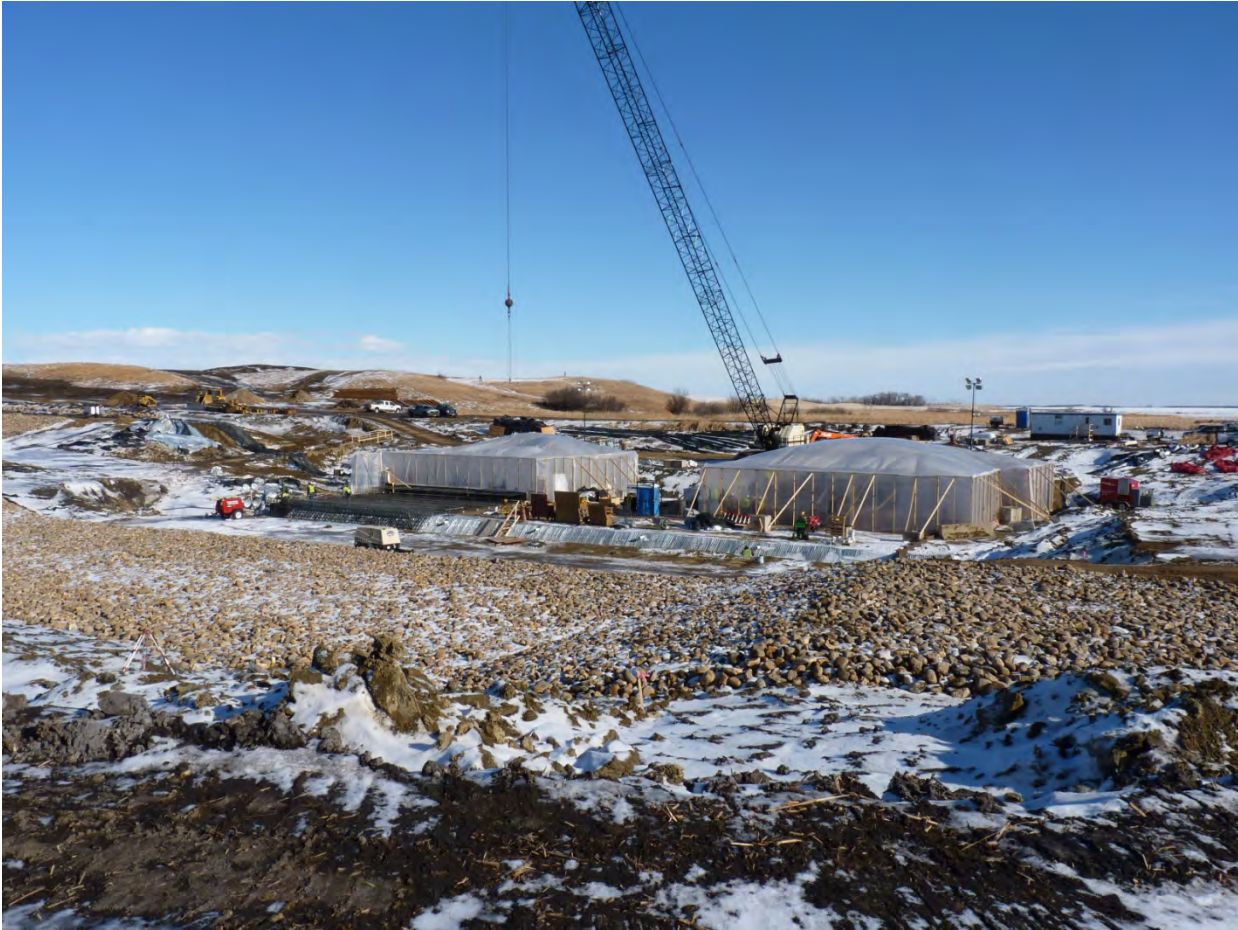
Figure 1: Photograph of Site
