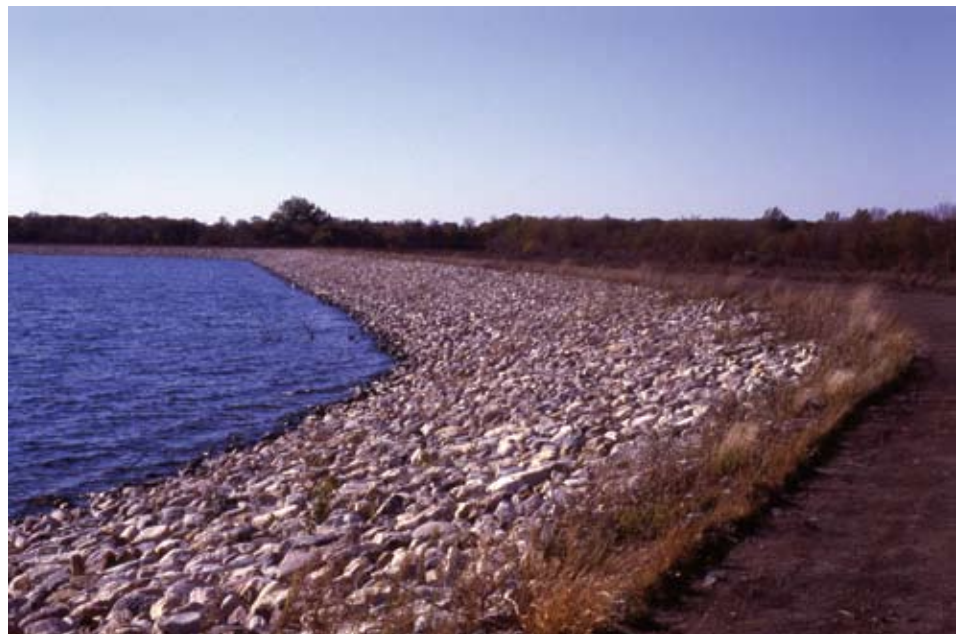
Figure 16. Protective dike, ground level. Photo by the author, October 6, 2004.
