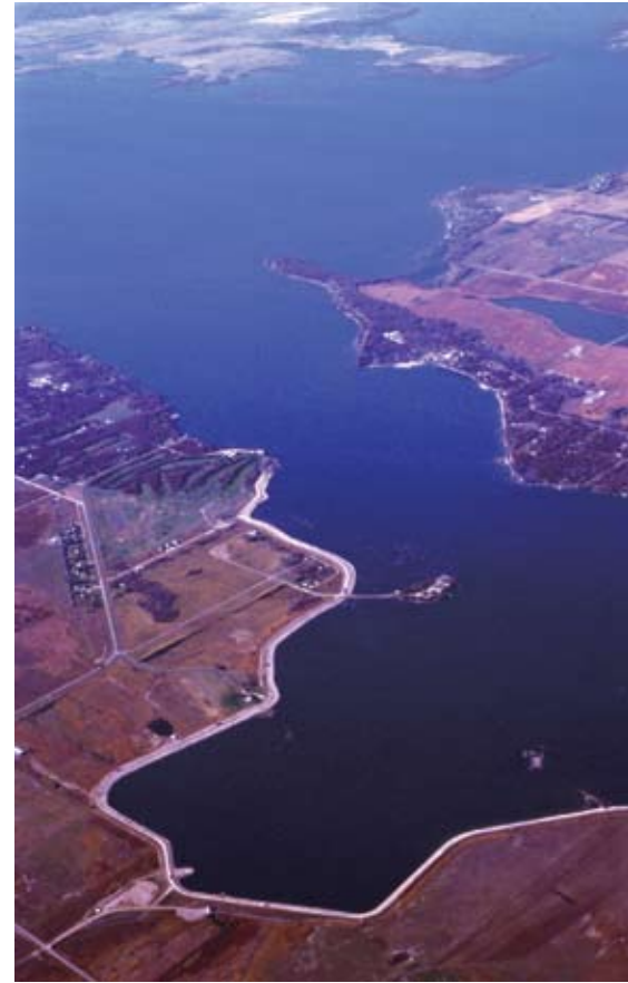
Figure 15. Aerial view of the City of Devils Lake and the protective dike. Photo by the author, October 9, 2004.
