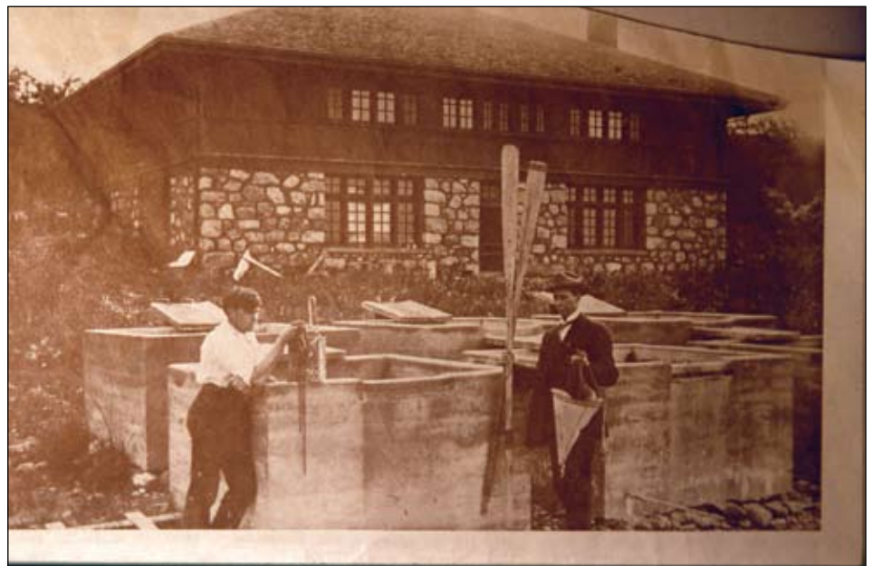
Figure 8. Researchers with equipment at the North Dakota Biological Station, circa 1914. In March 1995, as rising lake waters threatened to engulf the building, the upper half of the structure was lifted off the lower rock walls and moved to higher ground on the lake's south shore. Purchased by a private party, the building was restored and converted to a family residence. Photo taken by J.V. Harrison of Devils Lake, North Dakota.
